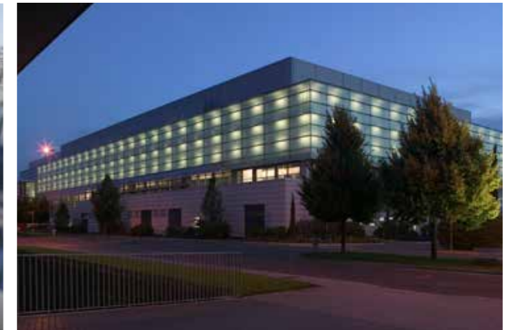
FERRARI PAINTSHOP BUILDING - MARANELLO (MO)
