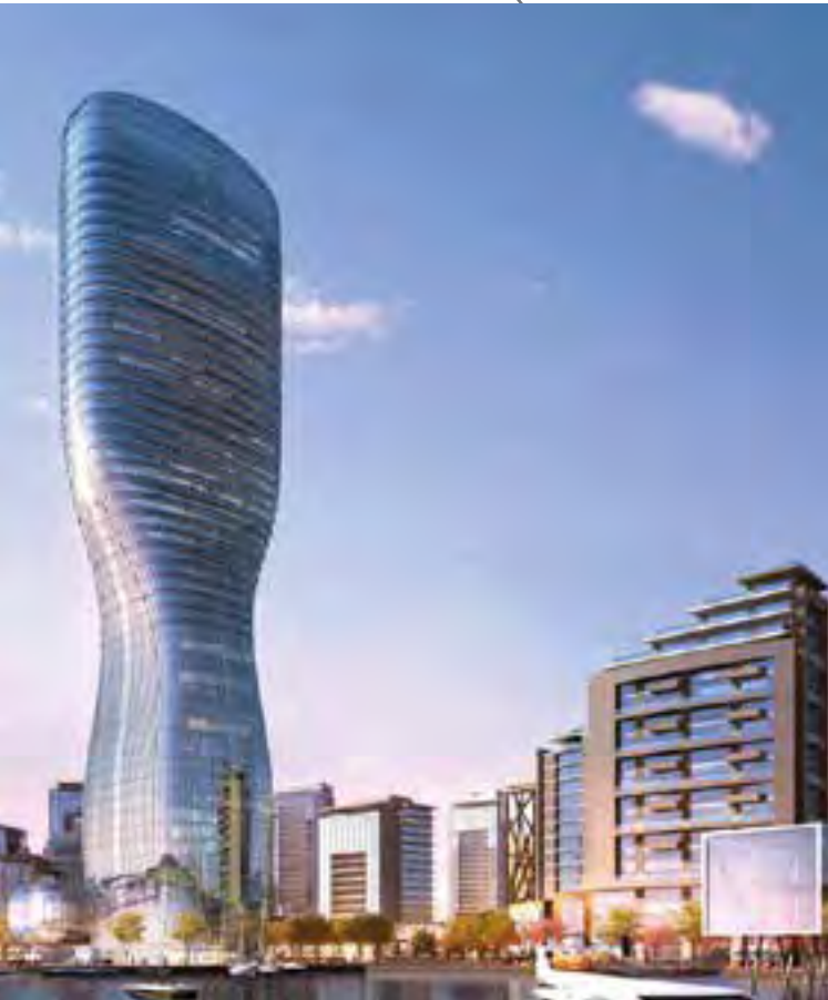
KULA TOWER - BELGRADE SERBIA - 2022 - Heating/cooling system
