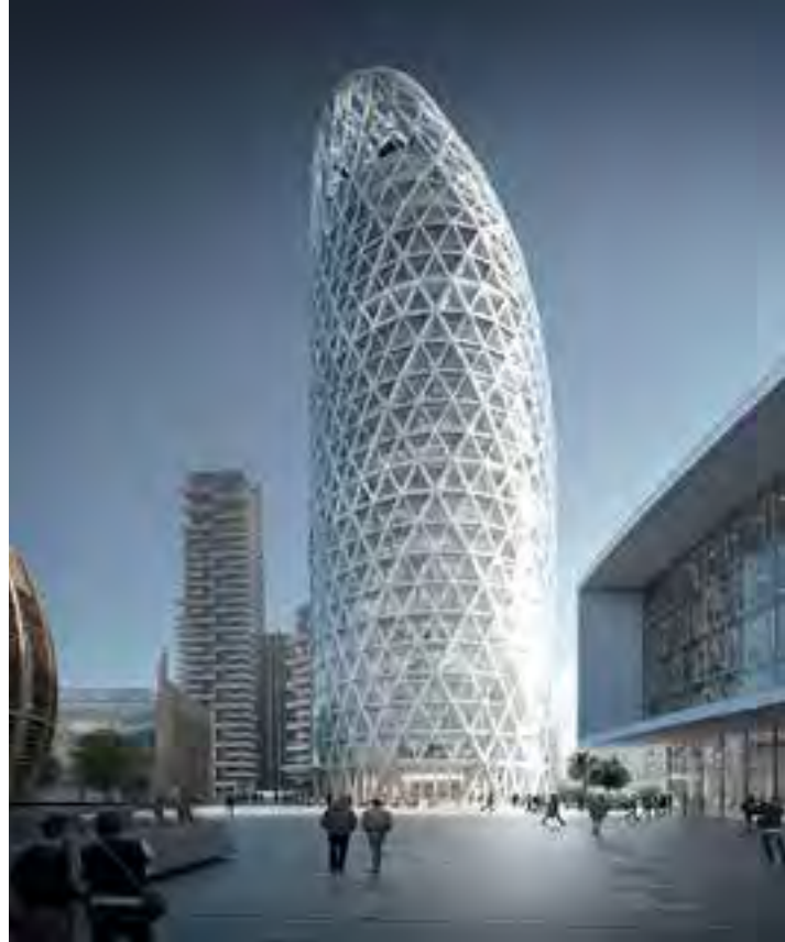
TORRE UNIPOLSAI - MILANO ITALY - 2023 - Central heating/cooling
