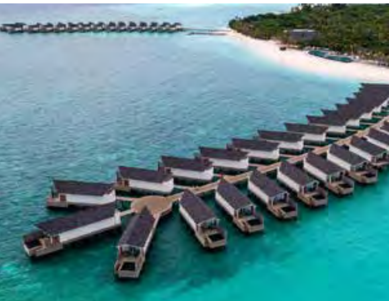
OZO RESORT - KUDAKURUTHU MALDIVES - 2021 - Water supply system
