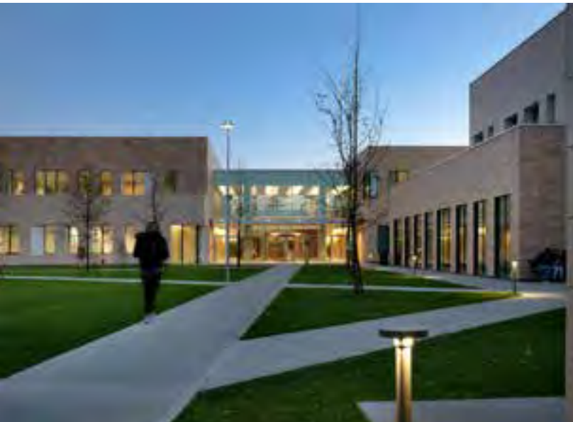
CAMPUS HUMANITAS - ROZZANO ITALY 2021 - Heating/cooling system
